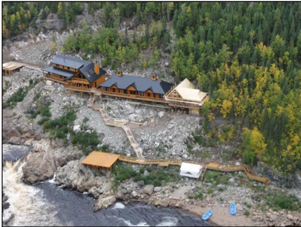
Figure 4: St. Lewis River Lodge
